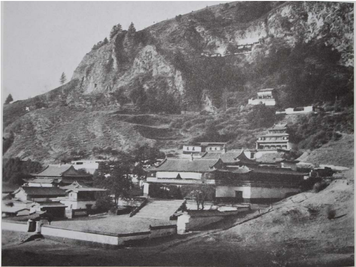
Gönlung in 1934. The main assembly hall and Changkya's villa are in the foreground. Photo by Zhuang Xueben. 74
