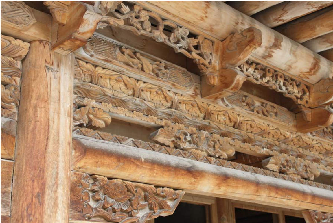
Detail of the woodwork of the Likya villa.
